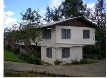
New residence in Mt Hagen
